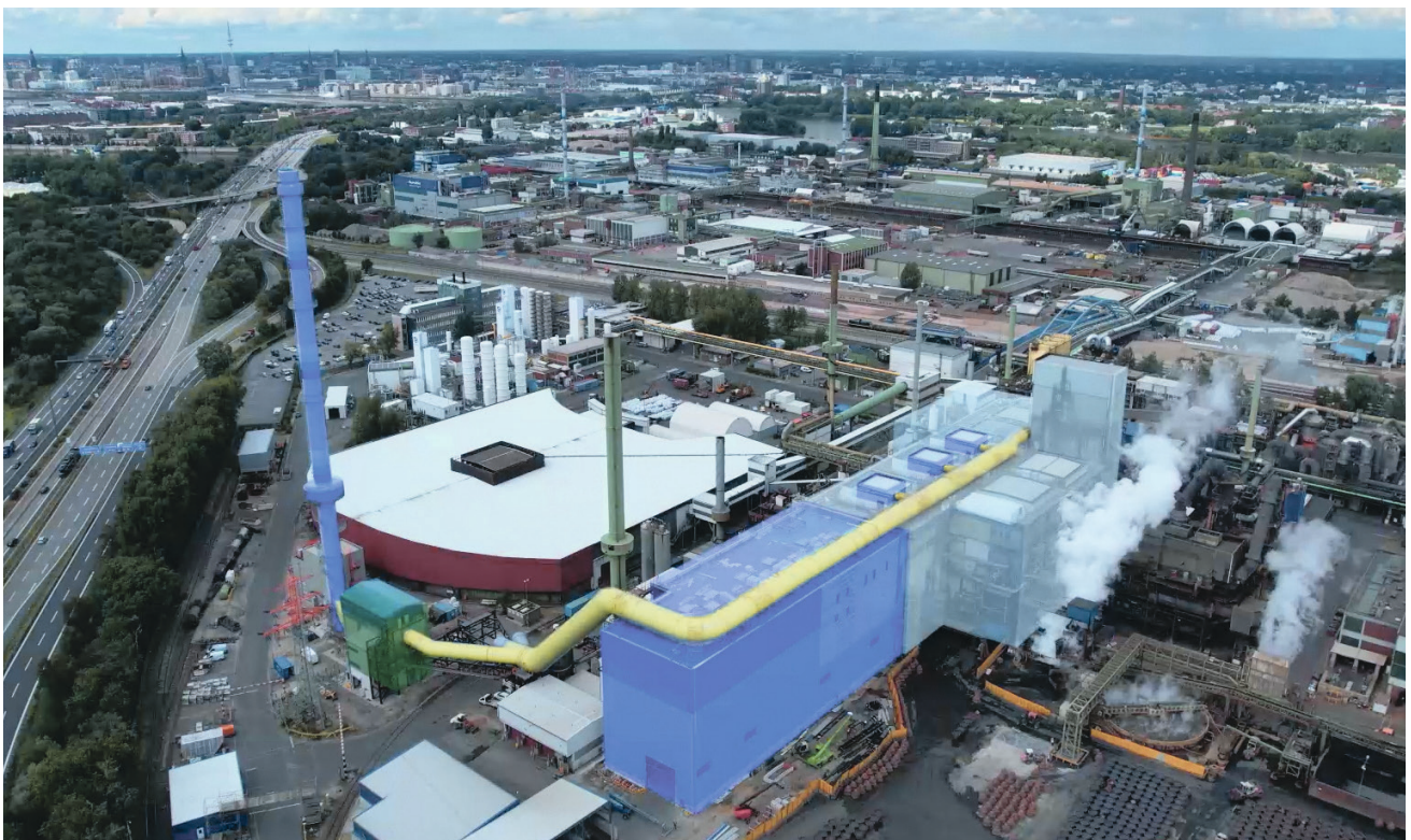
View of the new exhaust system (highlighted in color) at the Hamburg site in direct vicinity to the city
