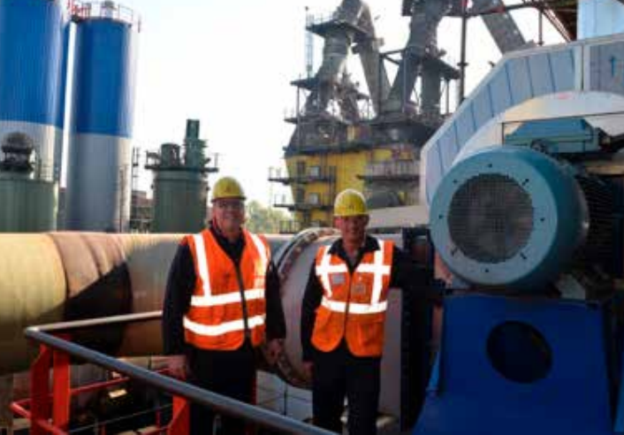
Planner Andreas Heuer and Plant Operator Carsten Holst in front of the fan of the new filter facility for concentrate drying, which was successfully commissioned in 2018.
