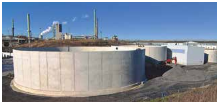
New rain retention basin at the Lünen site
