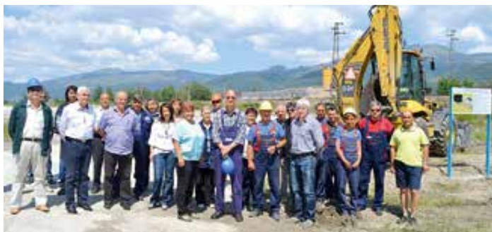
Start of construction of the water treatment plant at the Pirdop site
