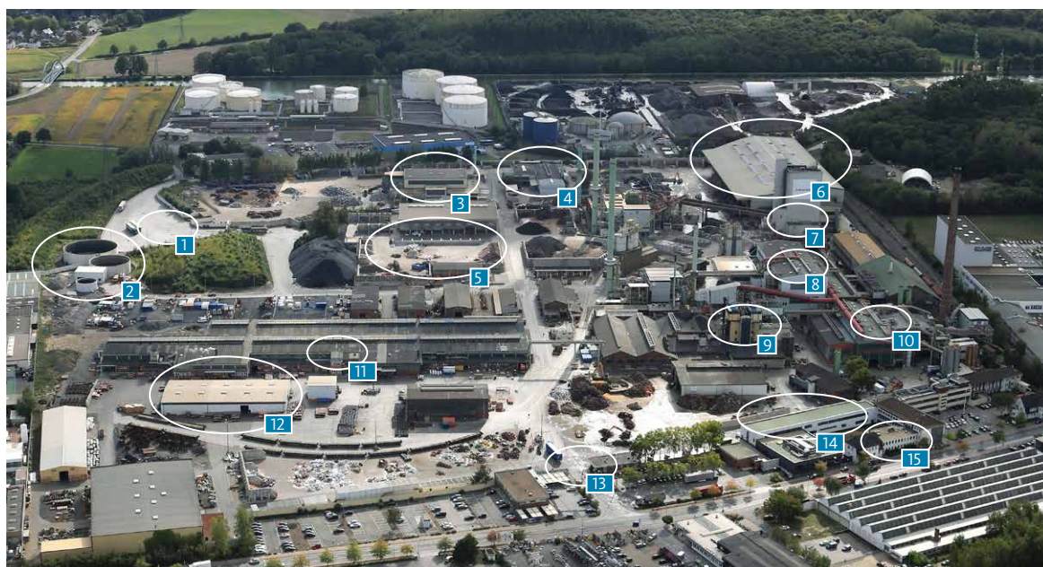
Fig. 3.1: Overview of Lünen site facilities
