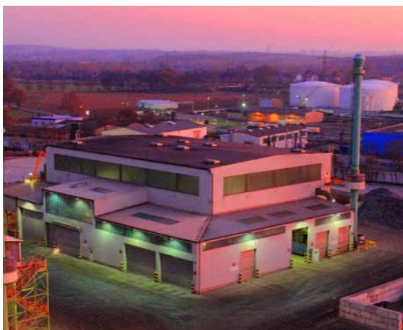
Aerial photo of the material preparation, crushing, and separation plant (MV-ZS facility) in Lünen
