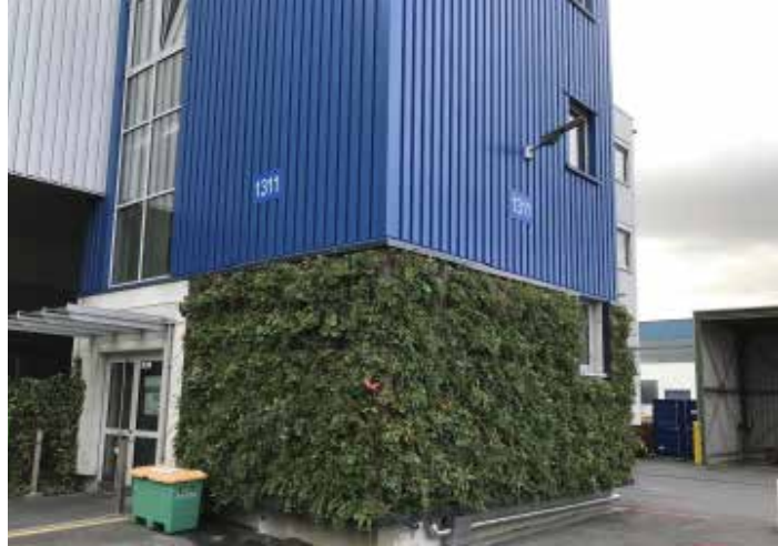
Adding greenery to vertical surfaces of an office and production building in the plant
