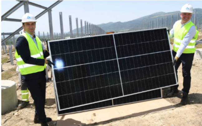
Groundbreaking ceremony for the photovoltaic system at the Pirdop plant on June 24, 2021, with Prime Minister Kiril Petkov and Aurubis CEO Roland Harings
